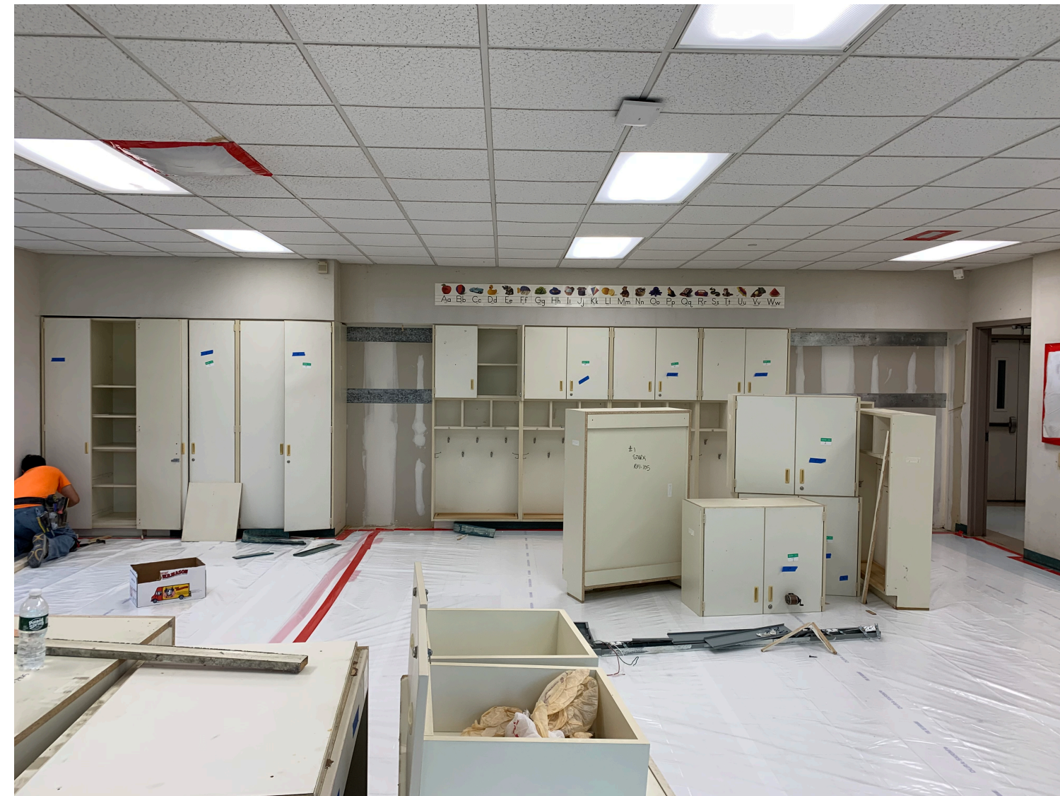
Room 105 removal of millwork
