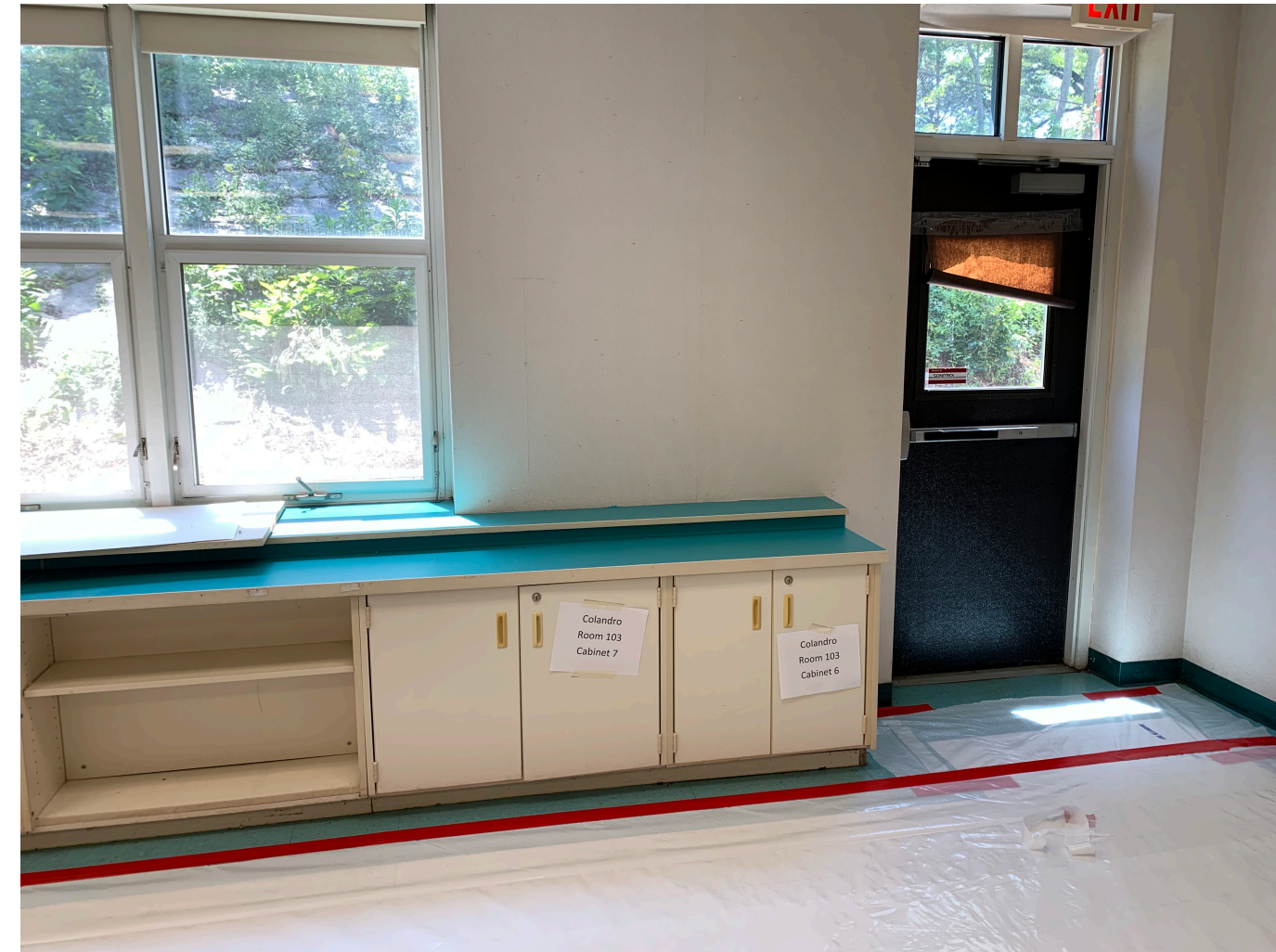
Room 103 Before beginning demo
