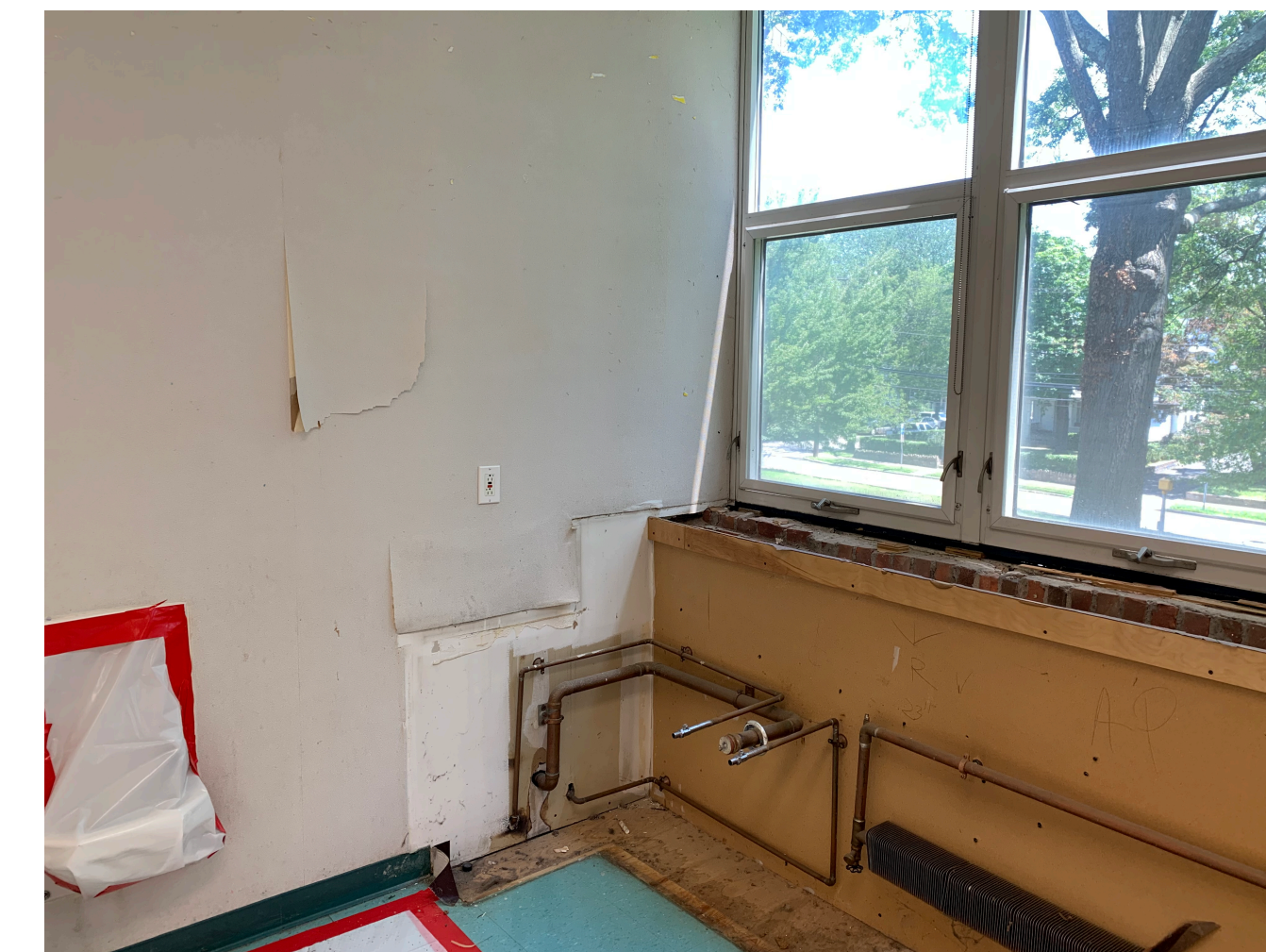
Room 105 removal of wall covering
