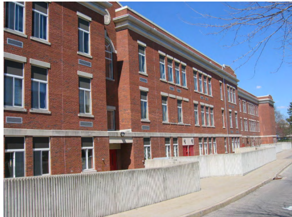
Photo #70: View of the rear façade. Note the flood barrier.
