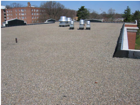
Photo #75: Second view of the main roof towards the north.
