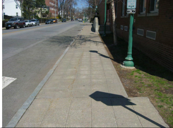
Photo #8: View of cast in place concrete sidewalks along Adams Street.
