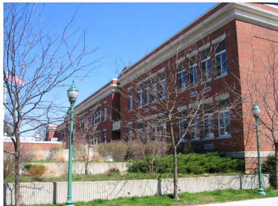
Photo #66: View of the front façade. Finishes of the exteriors are typically unpainted brick.
