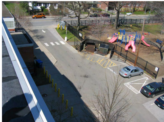
Photo #64: Overview of the north entrance driveway. No striped access aisle exists at main north entrance to playground.
