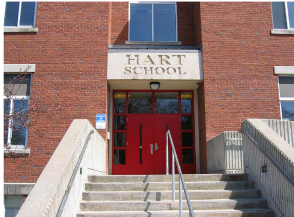
Photo #58: View of the main office lobby entrance.
