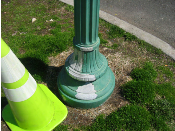
Photo #7: View of deteriorated paint coverings at the base of pole-mounted light fixtures.
