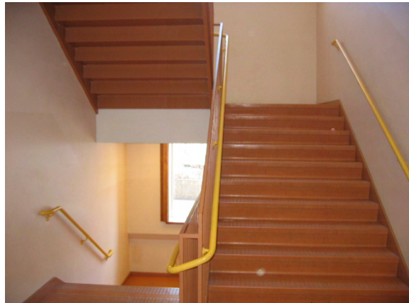
Photo #46: View of fire rated stairwell.
