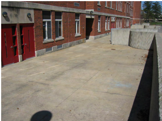
Photo #59: View of the rear main entrance. Note the flood retention walls.
