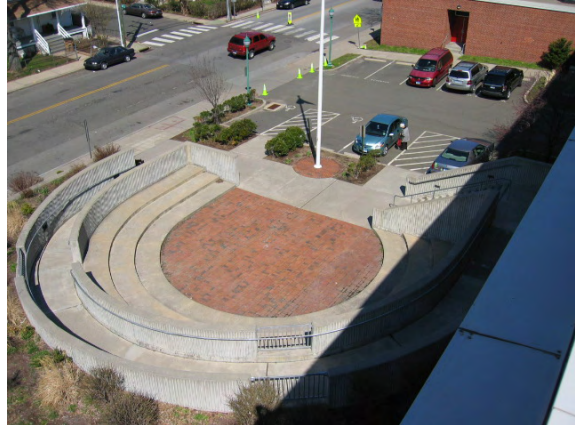
Photo #62: View of the circular concrete ADA wheelchair ramp at front entrance.
