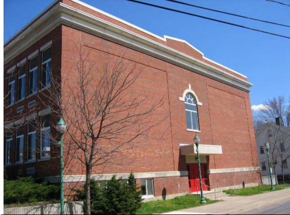
Photo #68: View of the south sidewall.
