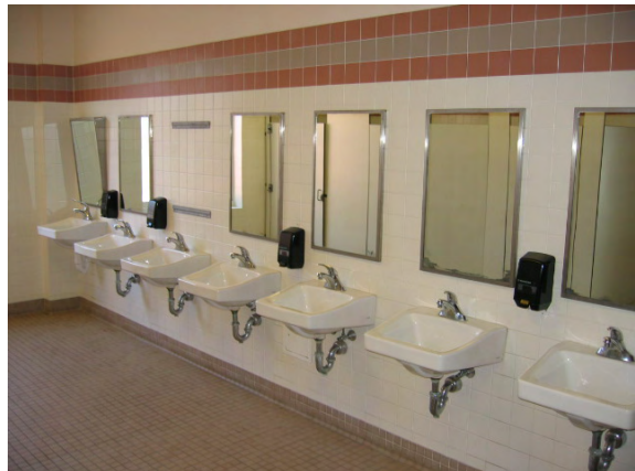
Photo #108: View of a typical ADA compliant multi-user toilet room.
