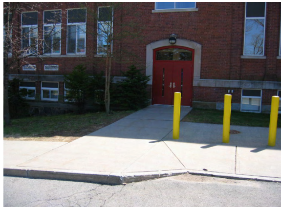
Photo #60: View of the north building entrance.
