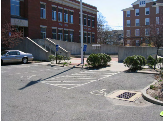
Photo #61: View of the handicapped accessible parking stalls at the front lot. Note missing posted sign to right.
