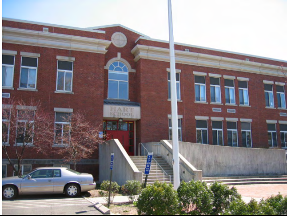
Photo #1: View of property identification signage.
