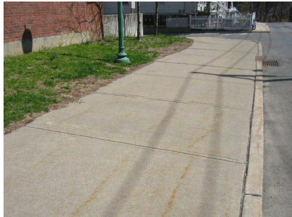
Photo #10: View of cast in place concrete sidewalks along Green Street.
